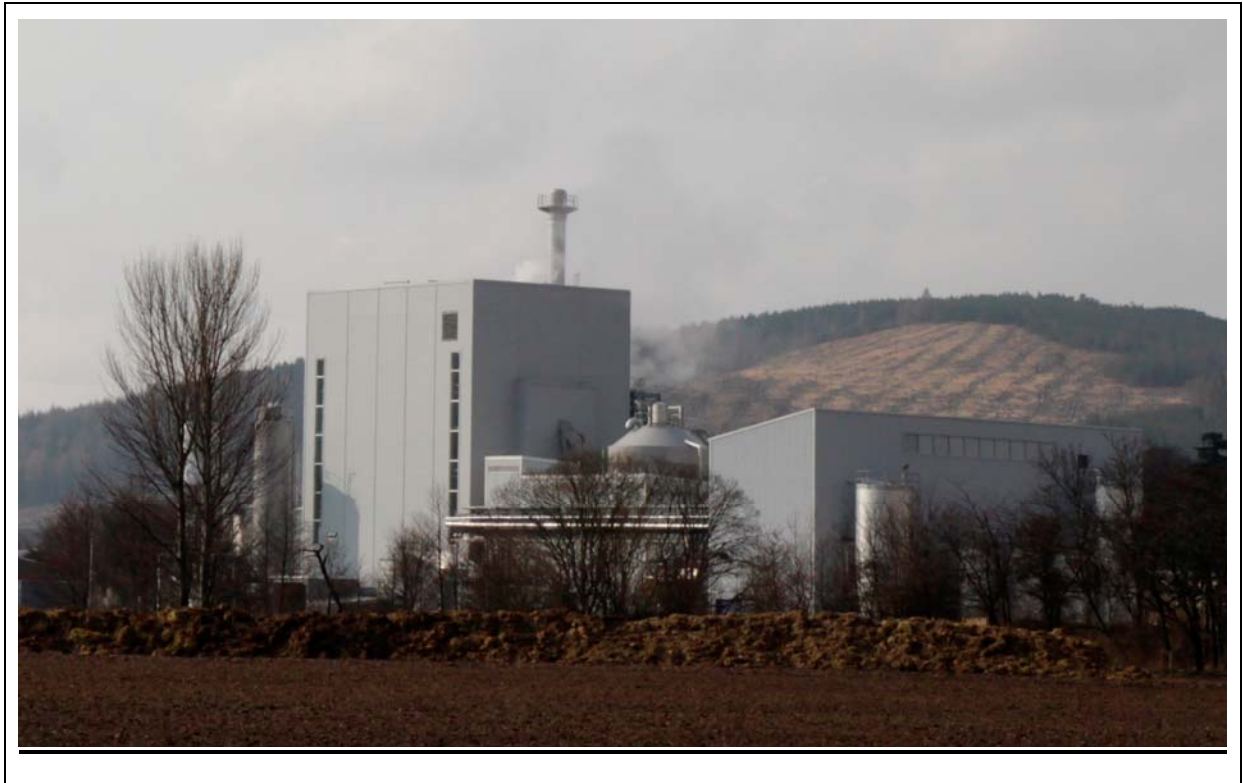
The Helius CoRDE biomass fired CHP plant at Rothies, Morayshire in Scotland.
